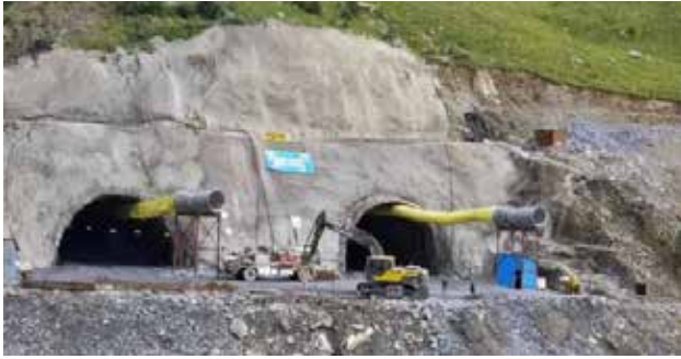
Construction Activity at Zojila Tunnel
